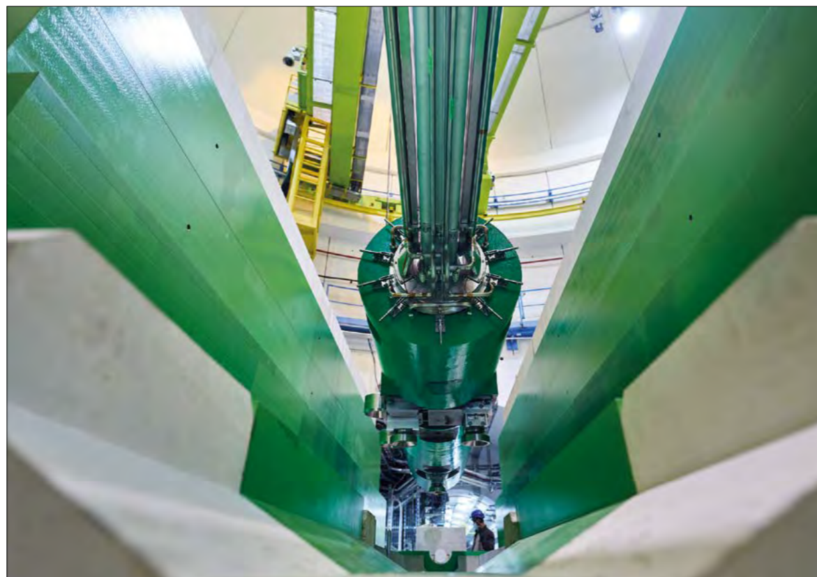
Structural integrity The new Super Proton Synchrotron internal beam dump being installed inside its shielding in October 2020.
