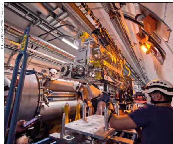
New collimators Left: new dispersion-suppressor collimators being installed near ALICE in 2020, where they will clean beam losses at the HL-LHC. Right: checks during collimator installation in one of the SPS-to-LHC transfer lines in November 2019, as part of the LHC Injector Upgrade Project.
